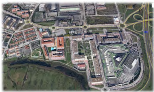
Nueva Montaña pilot zone where the Smart Water project was deployed.
