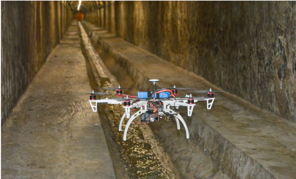
One of the drones used to perform sewer inspection tasks.
